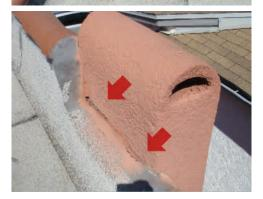
516 COMMENTS [CR] The roofing material and mastic /tar is separated from the left short cosmetic chimney.
