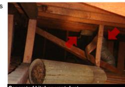
**602 COMMENTS** [SC] The kitchen vent duct is separated. This condition is potential a fire safety hazard.
