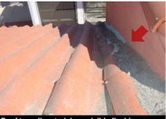
Roof to wall material, no visible flashing
