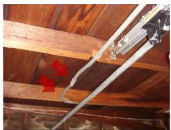
[CR] Areas of the framing has insect damage and moisture damage to the rear door jambs.
