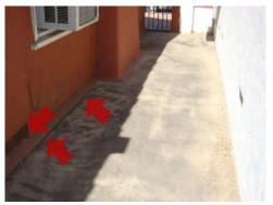
The house foundation adjacent to the the left sidewalk has excessive efflorescence from moisture. See picture 211 below.
