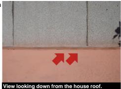
**401 EXTERIOR Description:** The low sloped roofing material has been updated with a suspected single-ply torch applied modified bitumen.
