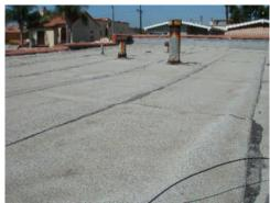
502 ROOF COVERING(S) Built-up roofing with a mineral surface cap sheet surface at the low sloped roof area.
