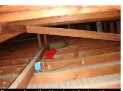
Romex wire spliced into knob & tube wiring
